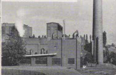
For miles, this 200-ft. chimney is a landmark
