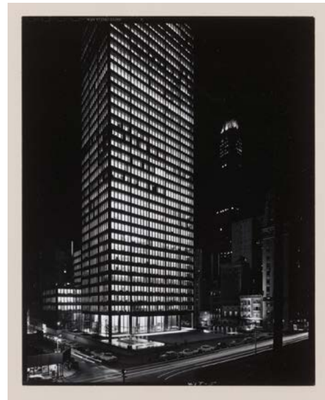
Partial view of the Seagram Building and plaza at night from across the street, New York City, 1958 or later. PH1990:0166. CCA Collection. © Esto Photographics, Inc.
